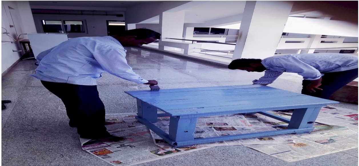
Termite Proof works for Water Cooler stand
